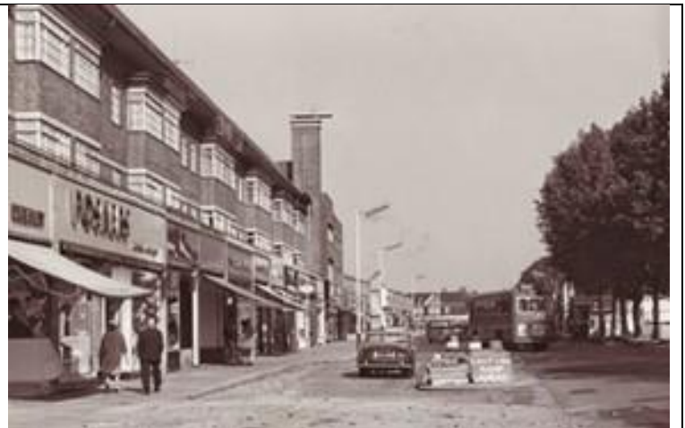
c1966 (widened High Street)
